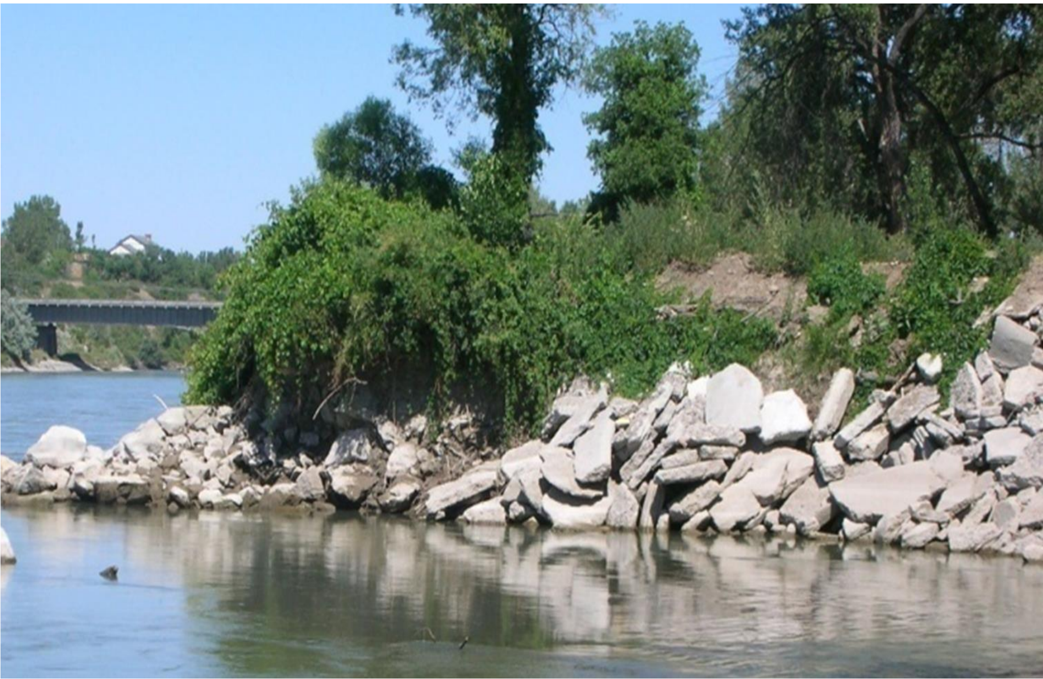
Figure 4: Residents using boulders as bank stabilization to minimize risk of erosion.
