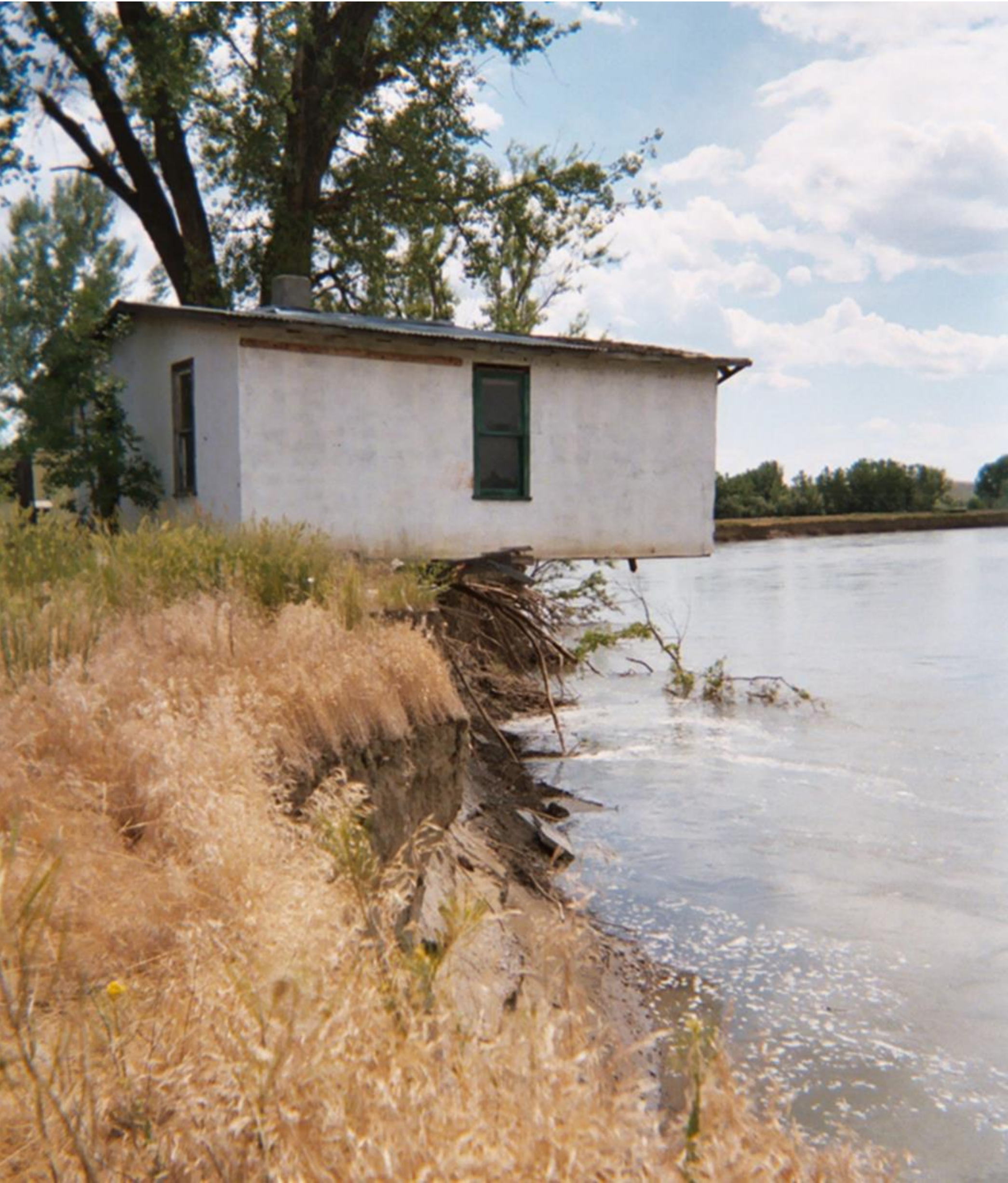
Figure 2: Impacts of erosion from annual flooding. Hysham, MT
