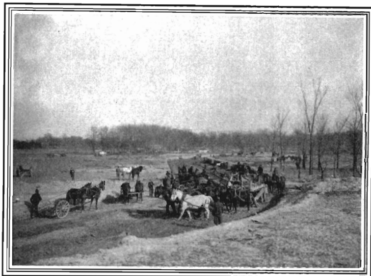
Grading a New Channel for River des Peres.
