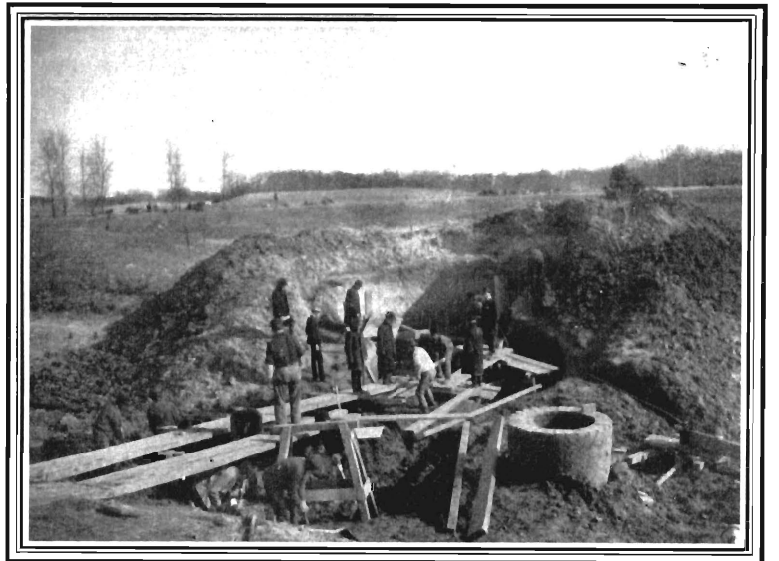
Pump Wells and Manhole for Sewer System.
