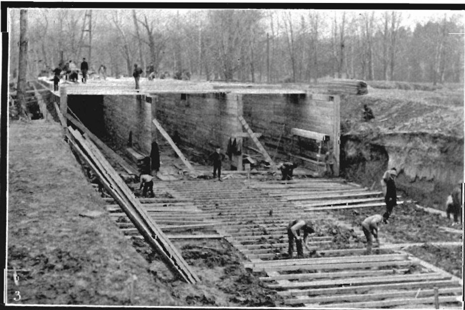
THREE STAGES IN CONSTRUCTION OF RIVER DES PERES CHANNELWAY. 1. Section of channel-way almost completed, showing floor, joists, uprights, and exterior backing. 2. Section of channel-way ready for the timber. 3. The advance work—packing clay between the foundation sleepers and sills.
