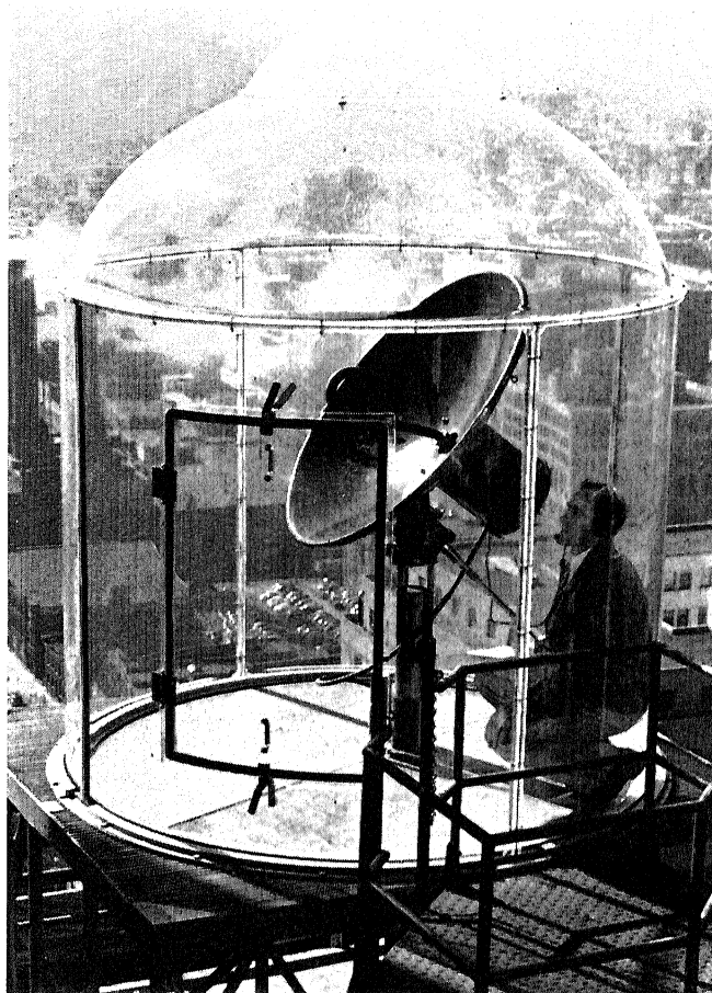
This plastic bubble atop the roof of Southwestern Bell Telephone Co. building houses television receiving equipment used in picking up telecasts from various points in the city and relaying, via video cable.
