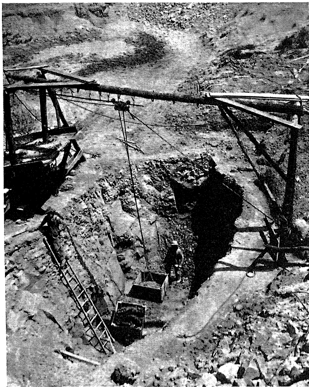
A. A type of hoist used in mining clay from deeper pits.
