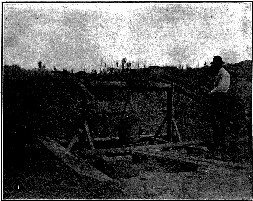
HAND WINDLASS HOIST IN OPERATION.
